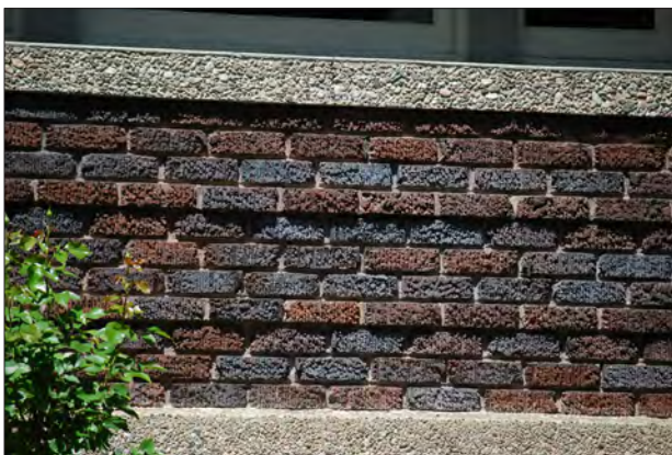
A decorative choice of materials, detailing and textures combines thermal mass with low maintenance.
