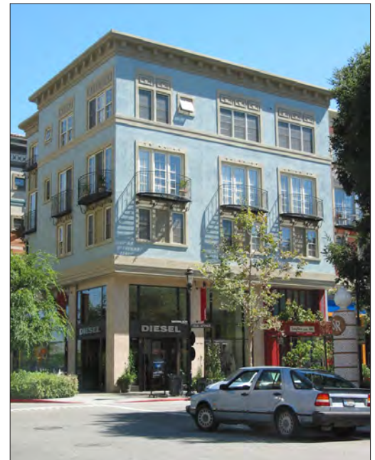
Window design and detailing here helps to identify the building's primary entrance on the corner.
