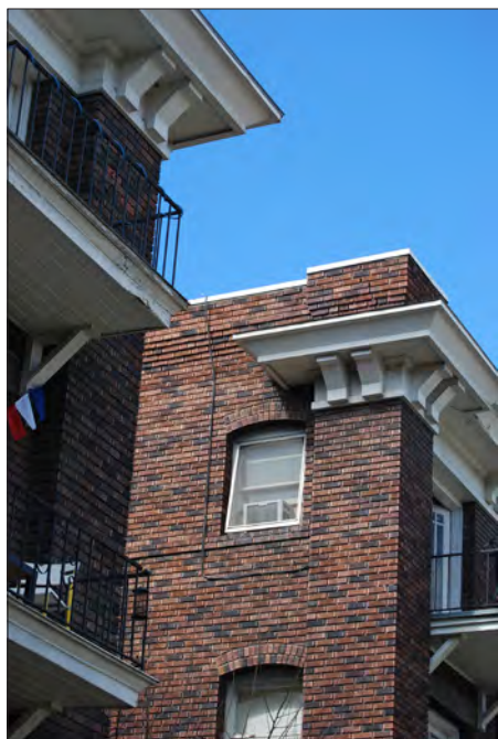
Cornice and balcony profiles and decorative brackets tie together the design detail of railings, windows and brickwork.
