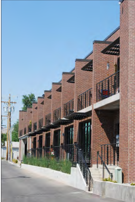
Contemporary multifamily development affording shaded private balcony space and first floor level windows.
