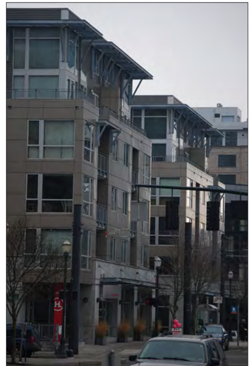
Symmetrical massing, emphasized by recessed vertical balcony bays, setting back top floors, and varied fenestration create both a distinct vertical proportion and sense of human scale.
