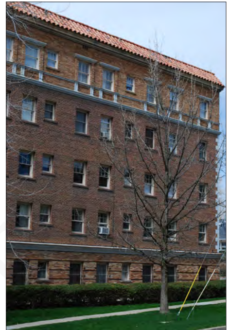
Differentiation in the design of the first floor and the top floor with tiled roof parapet help to frame the facade and reduce the perception of height.
