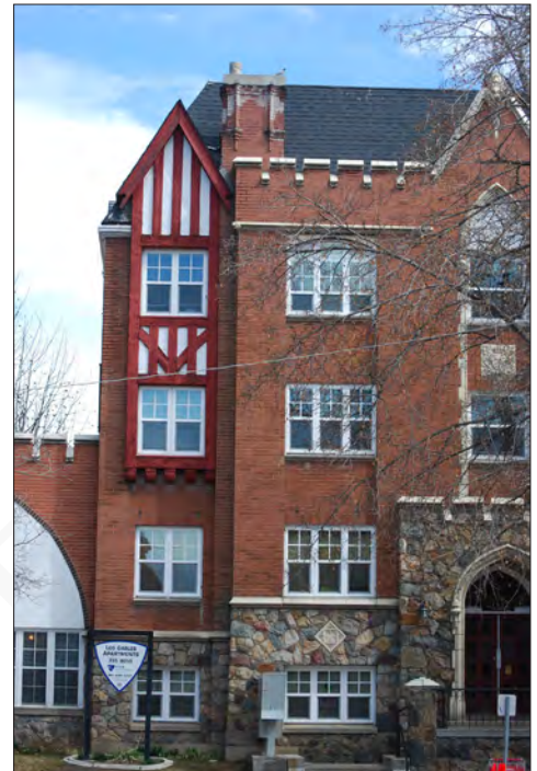
Symmetrical facade composition around a central entrance bay employs a change in wall plane, fenestration and gables to emphasize vertical proportion.
