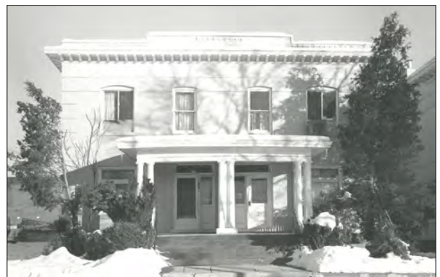
Four-Unit block, c. 1905, Salt Lake City, Salt Lake County. This elegantly proportioned, four-unit block of brick masonry has brick quoins and cornice with dentils below a short parapet. A portico of paired Tuscan columns protects the double entry to the building.
