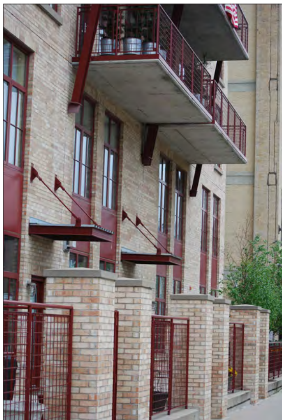
Dark red metalwork embellishes entrances, windows, railings and balconies within a brick facade, helping to convey the structural strength of the frontage.
