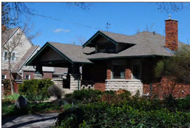
The architectural character of the building incorporates a variety of traditional design characteristics such as external porch, deep eaves, natural ventilation and solid masonry construction, ensuring efficient energy management and conservation.
