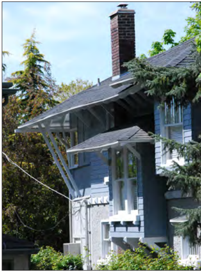
Projecting eaves provide protection from precipitation and solar exposure.
