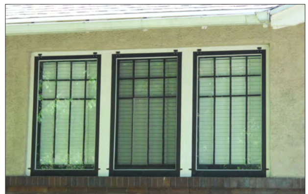
External storm windows combined with the original windows can outperform replacements in acoustic and energy terms.
