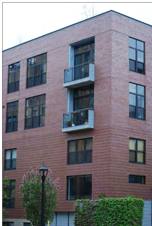
Metal window framing and textural detailing of the facade brickwork can achieve both visual strength and enrichment.
