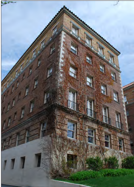
The design of the facade can effectively employ a hierarchy of windows reducing in stature on the upper floors, and establishing the actual or symbolic importance of levels and spaces.
