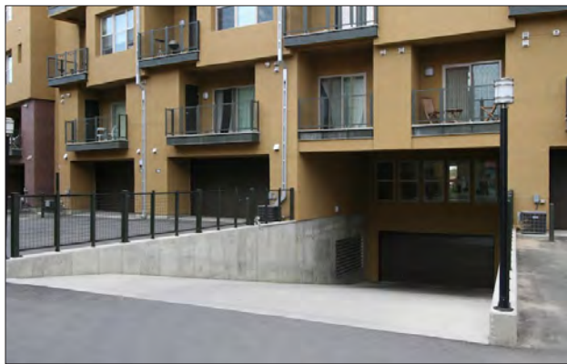
Vehicular ramped access is juxtaposed with street level garage entries, all situated to the rear of the building.
