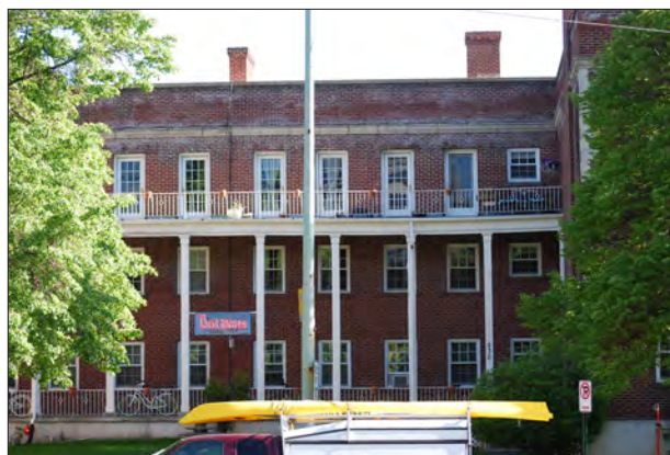
Bell Wines Apartments
