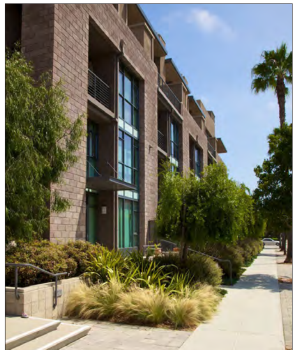
Integration of street facade and streetscape planting help to define the public from the private realm, and enhance both.
