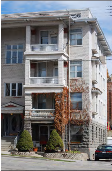
Window proportion and projecting balconies help to create a distinctive vertical emphasis.
