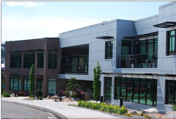
A contrast in facade design and materials, and the modeling of the facade can help to break down the lateral scale, while enhancing the visual interest and presence of the building.
