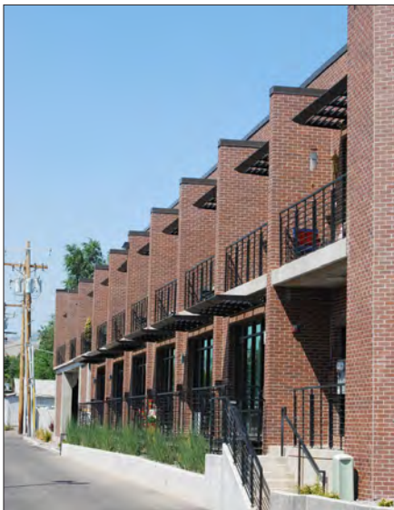
A linear sequence of of units stepping back to create strongly framed private balcony space above.
