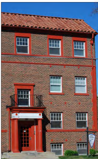
Clay roofing tile as a visible characteristic.
