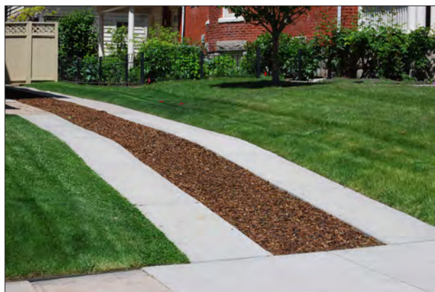
Drive strips or wheel strips are a historic solution to the contemporary issue of reducing impervious surface and runoff.
