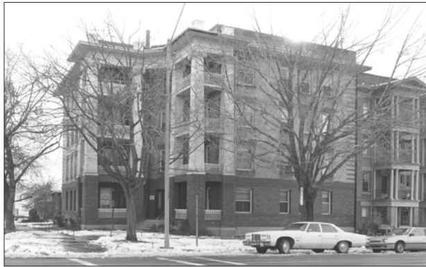
Apartment building, C. 1910, Salt Lake City, Salt Lake County. Another example of the “L” configuration, this block has a small forecourt at the corner of the lot. The projecting porches are supported, starting at the second floor, with tapered square Ionic columns that frame the corner entry.
