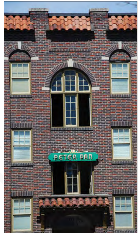
The considered detail inherent in the brick and tile work, as well as the window designs, create a vibrant street facade.
