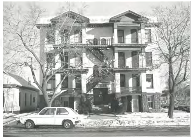
Rainer Apartments, c. 1900, Salt Lake City, Salt Lake County. The raised basement of this building helps create a sense of verticality characteristic of this apartment type.
